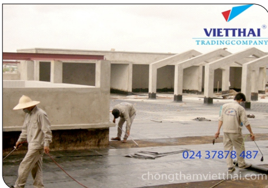
Construction of torched on membrane
